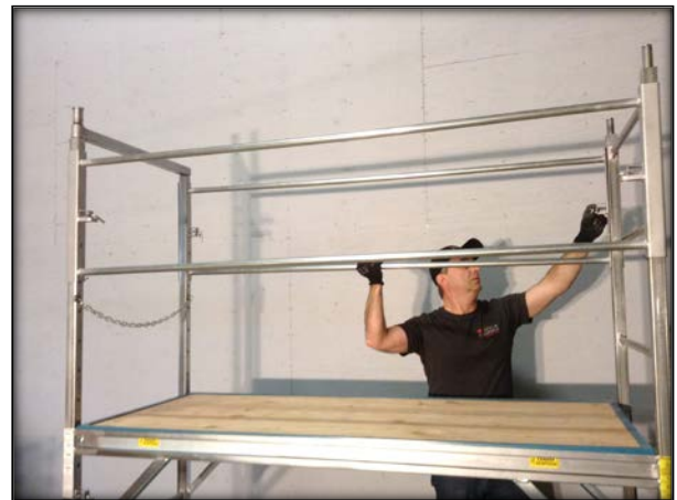
12B) Install back Guardrail second.
