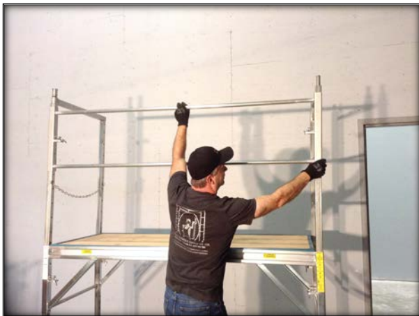
12A) Install front Guardrail first.
